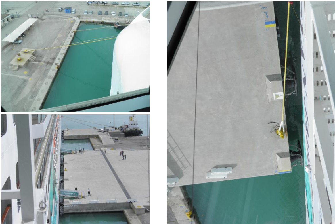
Figure 26. View from the supervision position at port bridge wing at Katakolo Port
